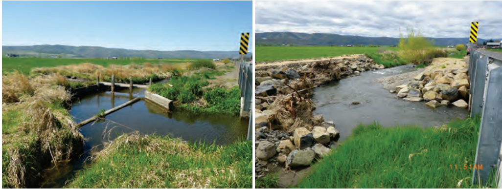
Irrigation diversion replacement (before and after)
