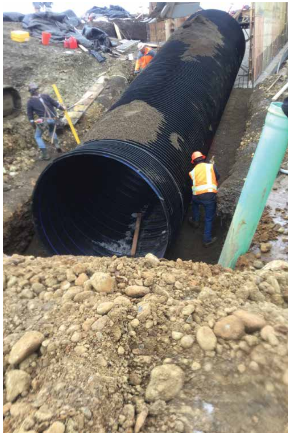
Crews work to install the 96-inch diameter pipe for the canal to pass under Coleman Creek.
