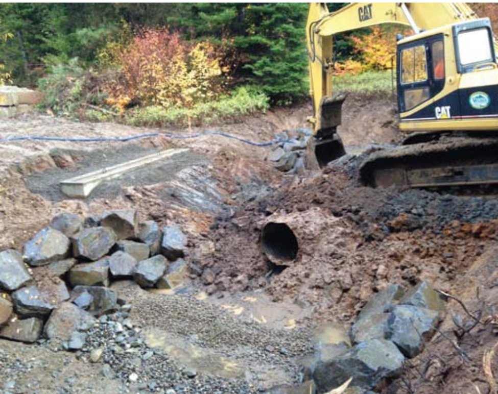
Removing the old, undersized culvert in preparation for the new bridge.
