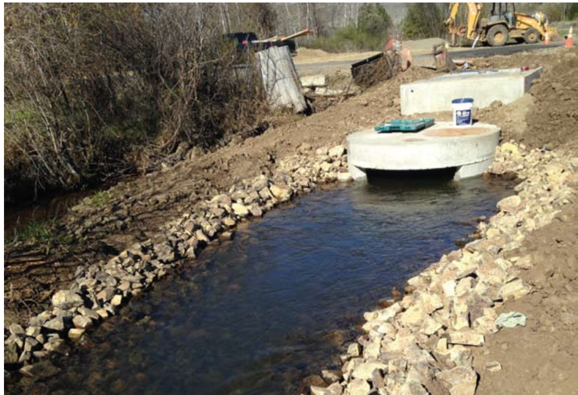
Pipeline outlet into Reed Ditch at Cove Road.
