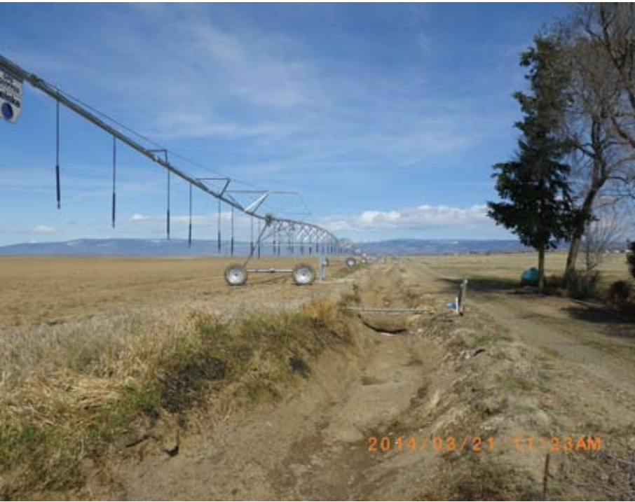
A new center pivot sprinkler system installed on 120 acres southeast of Kittitas.
